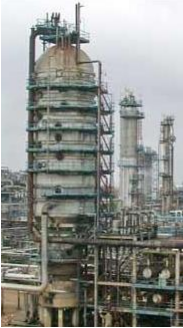
Large-scale, industrial vacuum distillation column [27]
